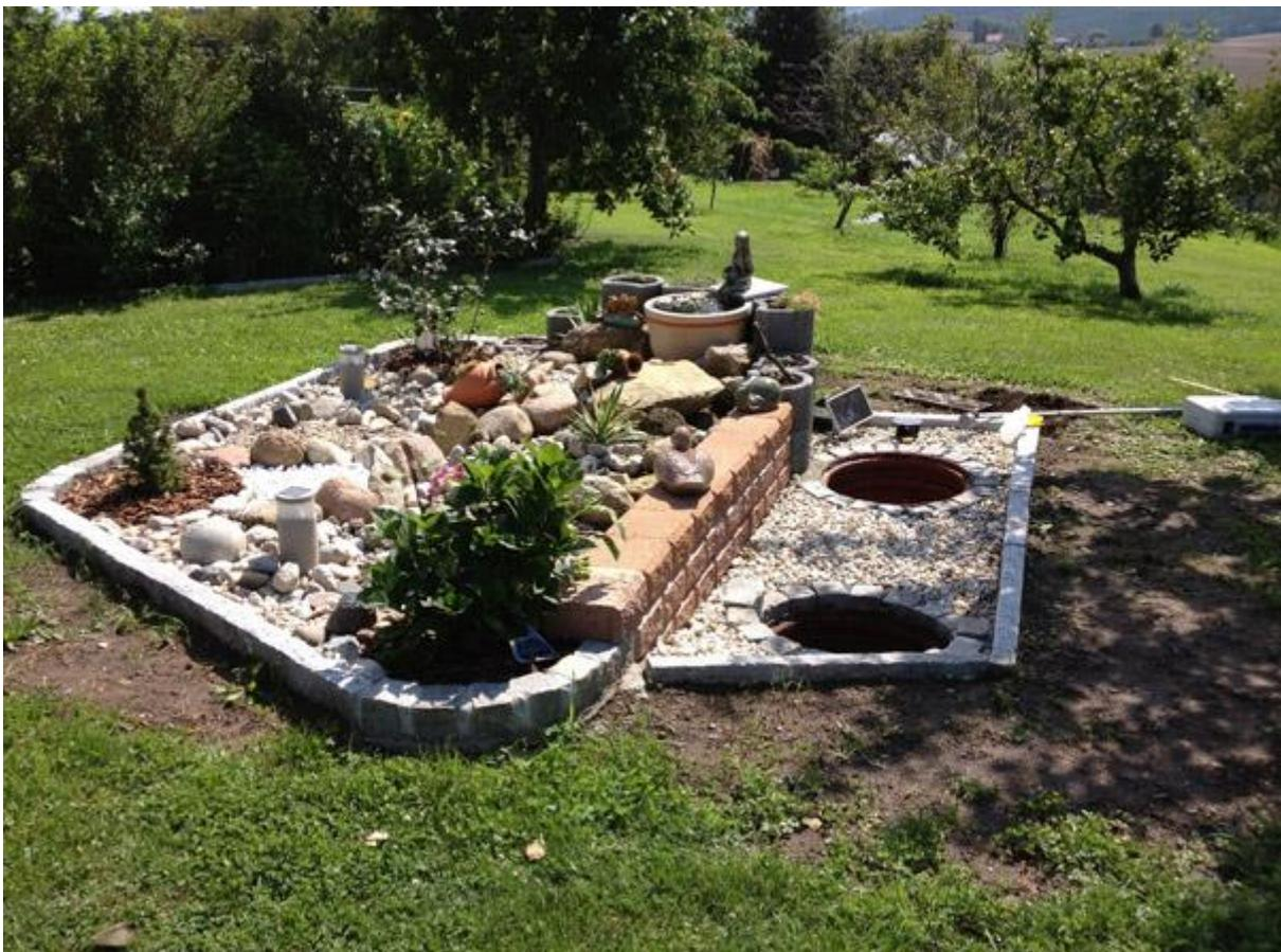
The picture shows a 4 p.e. ClearFox® nature treatment plant whereas the maintenance has been done, samples have been taken and the function of the system has been checked. The powerless ClearFox® nature system needs to be maintained every half year in accordance with other small wastewater treatment systems.
