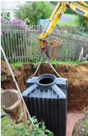
Installation of the small wastewater treatment plant with a small scale digger
