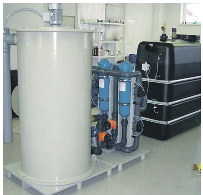
ClearFox® TBZ with reuse water tank up to 40m 3 /h
